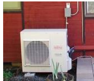
Ductless, Residential Heat- Pumps and Air-Conditioners
