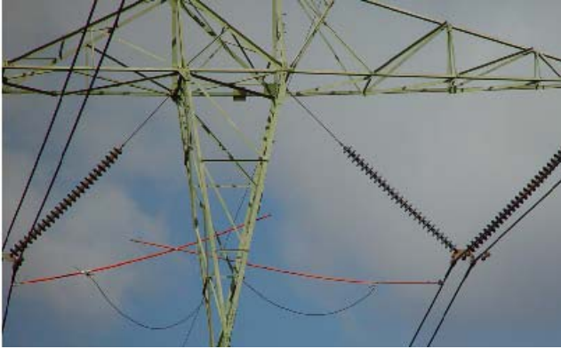
PPAGs installed on a 500 kV line.
