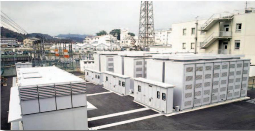
*Sodium-sulfur batteries, offered commercially under the trade name NAS, have shown great promise for utility applications in the 1–6-MW range. Based on a high-temperature reaction between sodium and sulfur, the NAS battery features excellent stability, robust cycling, and minimal on-site maintenance. Shown is a 6-MW unit installed at a substation in Ohito, Japan.*
