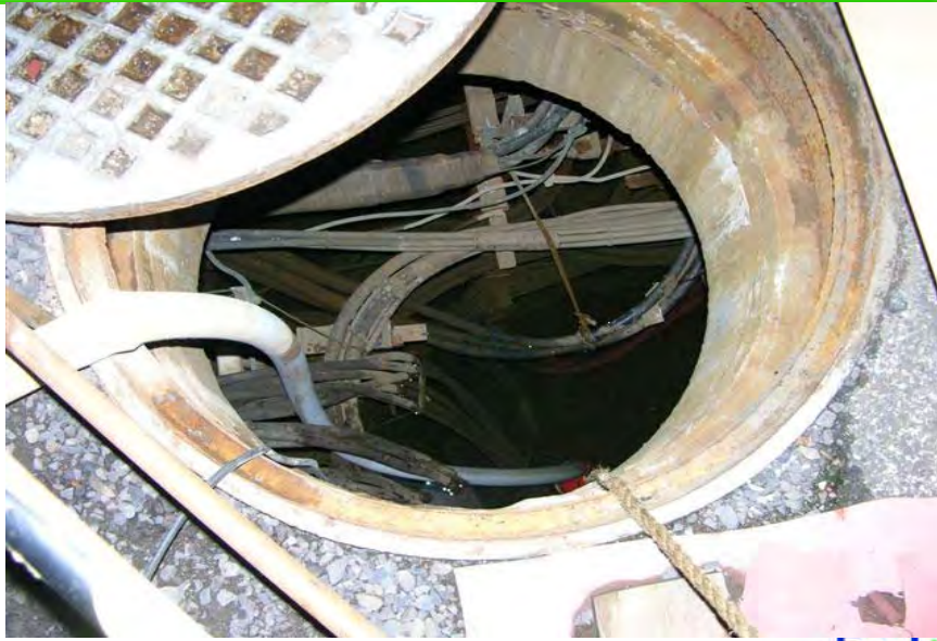
Manhole Containing Cable
