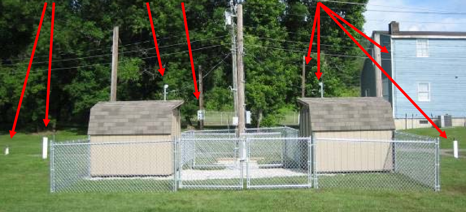
Previous Stray Voltage Testing Structure
