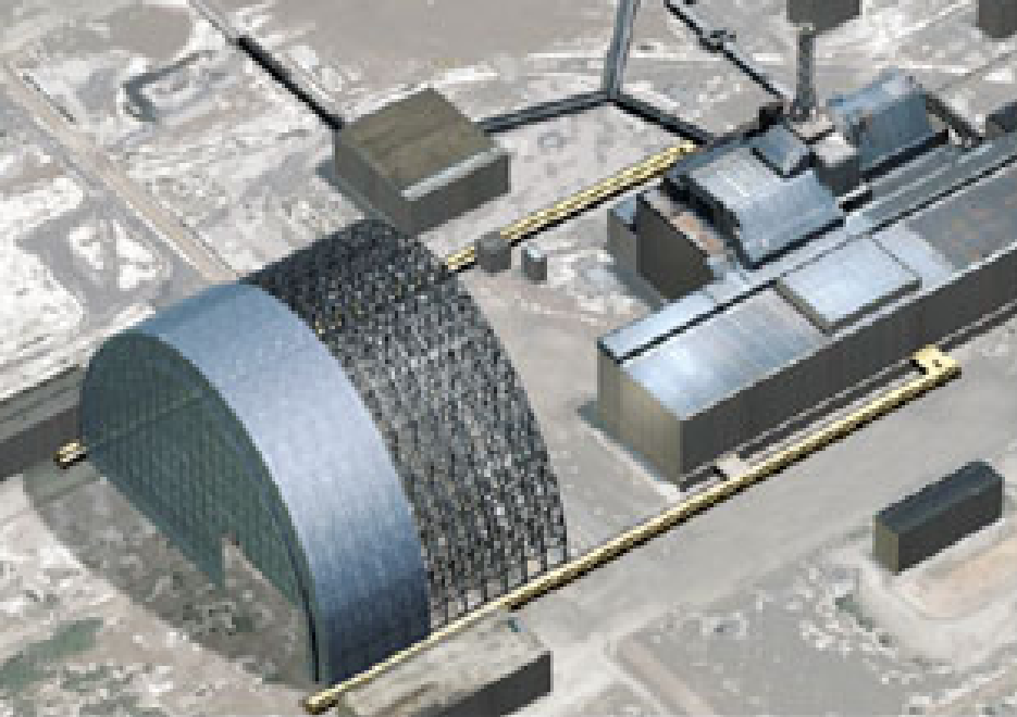
1) CONSTRUCT STEEL CASING NEAR REACTOR NUMBER FOUR
