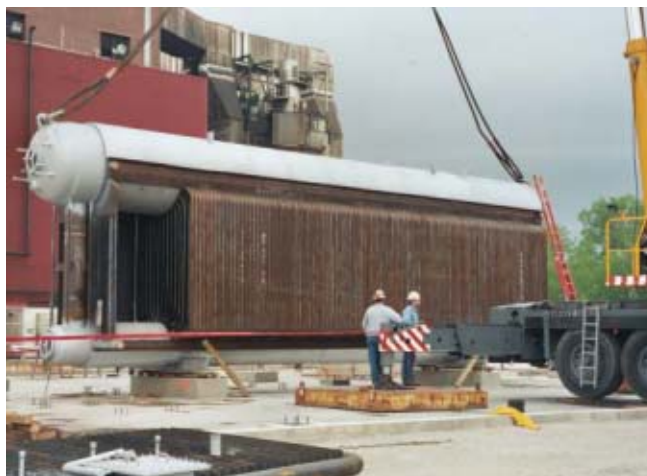
A modular boiler prior to being lifted into place. Photo courtesy Rentech Boilers.
