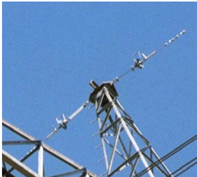
Ground wire configuration
