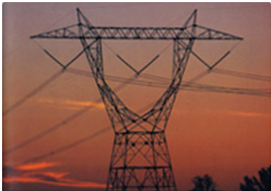
A 765-kV transmission line
