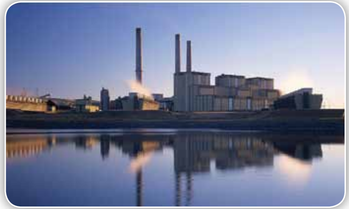
Tri-State Generation and Transmission Association's Craig Station
