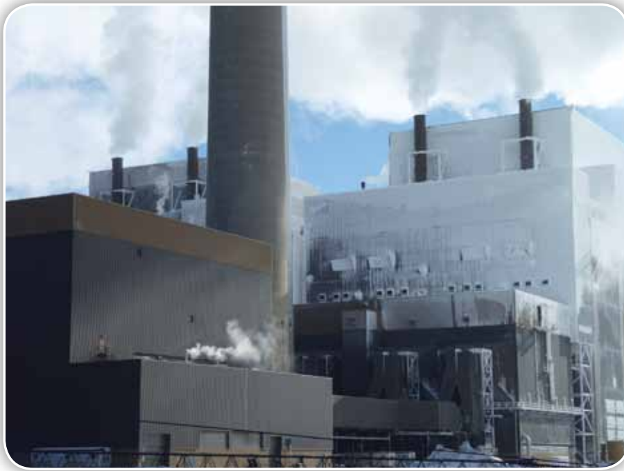
Had it not been removed from the coal, the water vapor leaving the DryFining™ system stacks at the Coal Creek Station would have become flue gas and added to the plant emissions.
