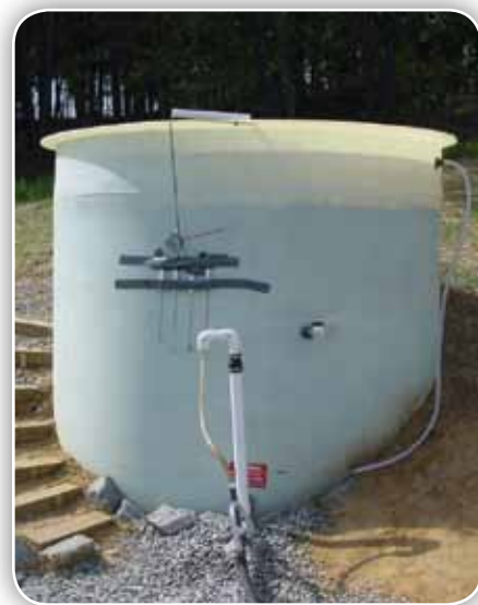
Pilot-scale vertical flow wetland
