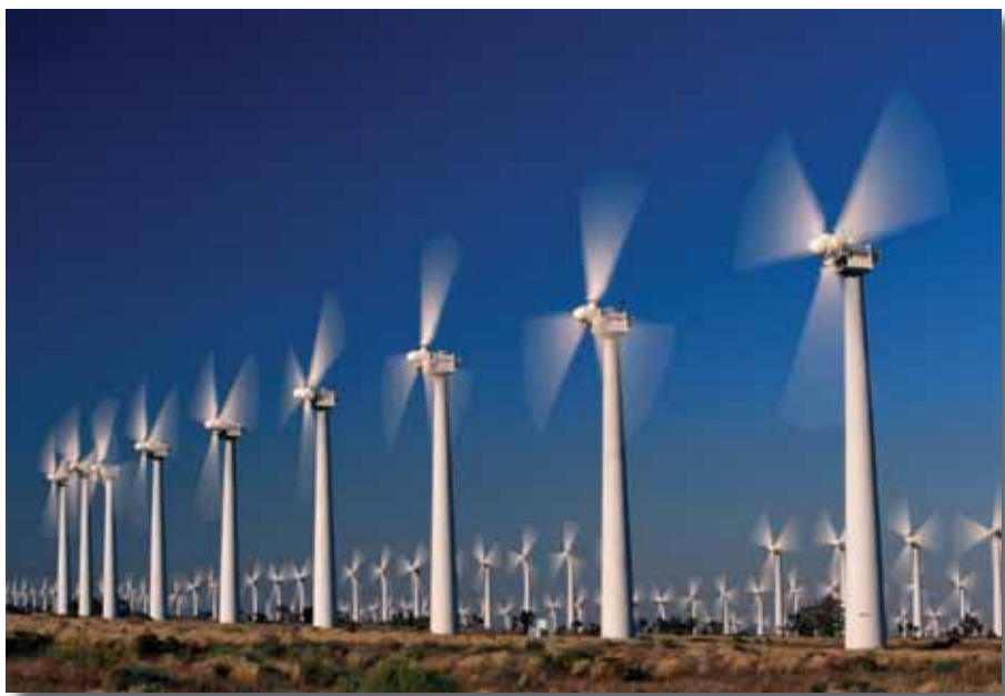
Wind power is now competitive with conventional electricity generation in favorable locations. Much of today's research is focused on dealing with the intermittency of the wind resource and integrating often-remote installations into the power grid.
