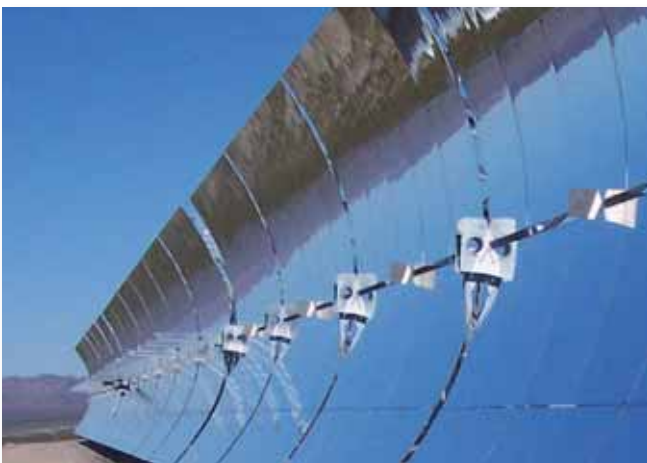
Parabolic trough systems are considered the most reliable and least costly of today's solar-thermal electricity (STE) technologies. The Nevada Solar One plant—a 64-MW installation that lines up 760 parabolic concentrator arrays—began generating power in June. (photo: Acciona Group)
