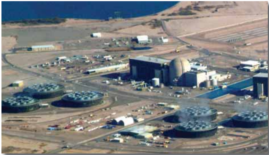
The Palo Verde nuclear generating station near Phoenix has been using treated municipal effluent—so-called gray water—to meet its plant cooling needs for over 20 years. The effluent is stored on-site in a 760-million-gallon lined reservoir.
