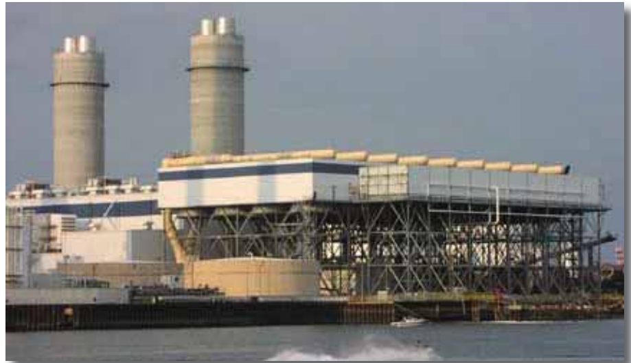
Dry cooling has obvious advantages in water-constrained regions but may be a good choice elsewhere as well. For example, the Mystic generating station on Boston Harbor chose a dry system over once-through cooling to avoid concerns over possible impacts on aquatic life.
