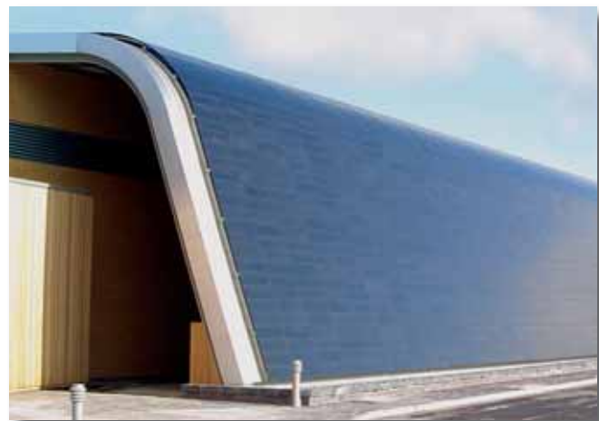
Thin-film photovoltaic cells, manufactured by depositing semiconductor materials on an inexpensive substrate, can be integrated with conventional building materials such as roofing tiles. In this 85-kW installation, CIS PV cells form an entire side of a business center in Wales. (photo: Shell Photographic Services, Shell International Ltd.)
