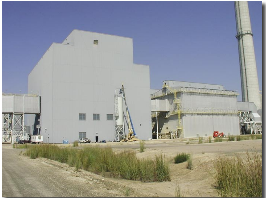
Sunflower Electric's Holcomb Station near Garden City, Kansas, was host to a full-scale field test of sorbent injection for mercury capture under the DOE-NETL program. Conventional sorbents injected into the flue gas duct (far left) before the plant's spray dryer unit achieved only modest results in removing mercury. However, use of a new, chemically enhanced sorbent removed 90% of the mercury at low-to-moderate injection rates. The sorbent is collected by the plant's fabric filter, and the cleaned flue gas exits the stack at right. (Photo courtesy ADA-ES)
