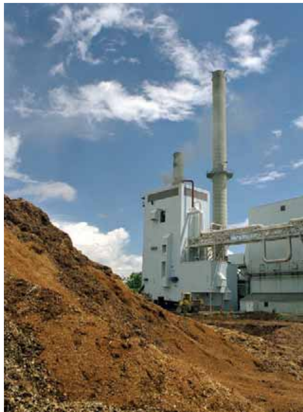
Wood chip residues from Vermont forests and sawmills supply the bulk of the fuel for Burlington Electric Department's 50-MW McNeil generating station. Biomass can be fired directly, as at McNeil, or gasified before combustion for very low emissions. (photo courtesy National Renewable Energy Laboratory)
