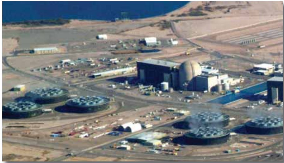
The Palo Verde nuclear generating station near Phoenix has been using treated municipal effluent—so-called gray water—to meet its plant cooling needs for over 20 years. The effluent is stored on-site in a 760-million-gallon lined reservoir.
